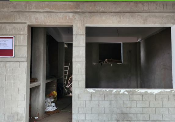
Kitchen shell is ready
