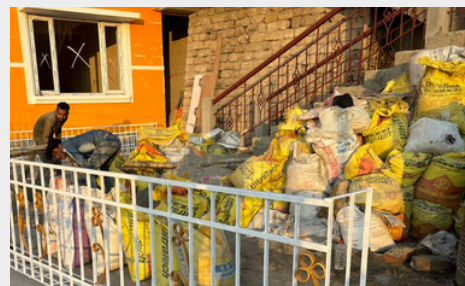
Stairs being made safe
