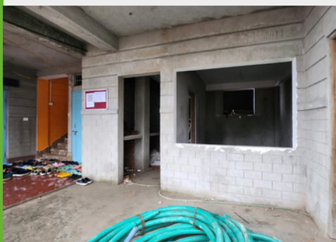
Completion of wiring & fitting gas pipes
