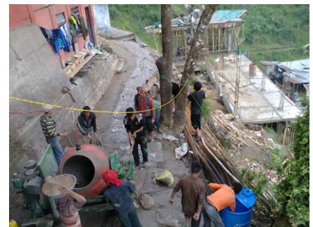
Concrete mixer and new buildings
