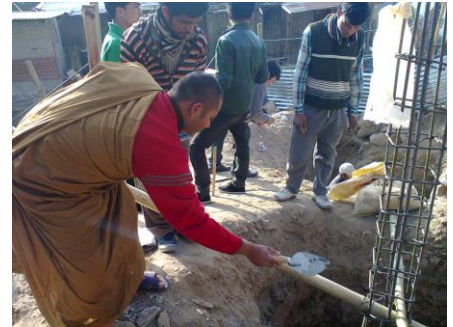
Pema Bhante lays the first concrete
