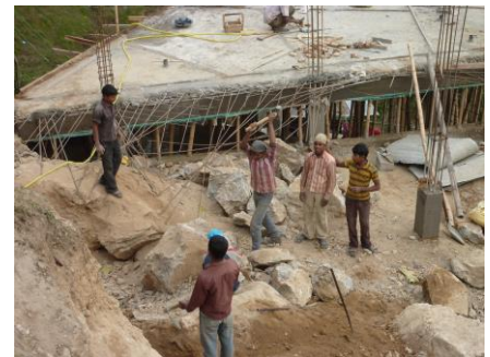
Breaking rocks manually
