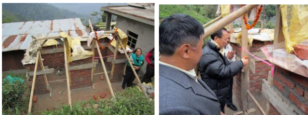
Toilets under construction and cutting the ribbon
