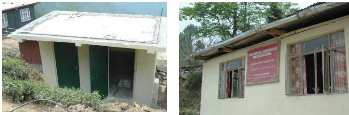
New toilets and windows.
