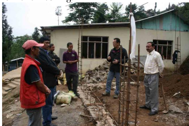
Discussions taking place at the school with staff. The glassless windows are clearly visible.
