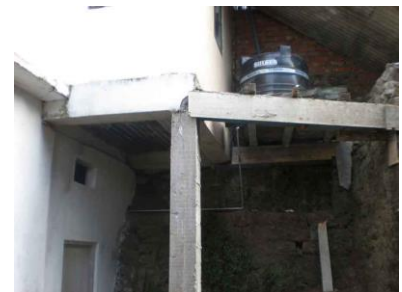
Water harvesting tank in place, Serotam located on concrete structure behind teachers.
